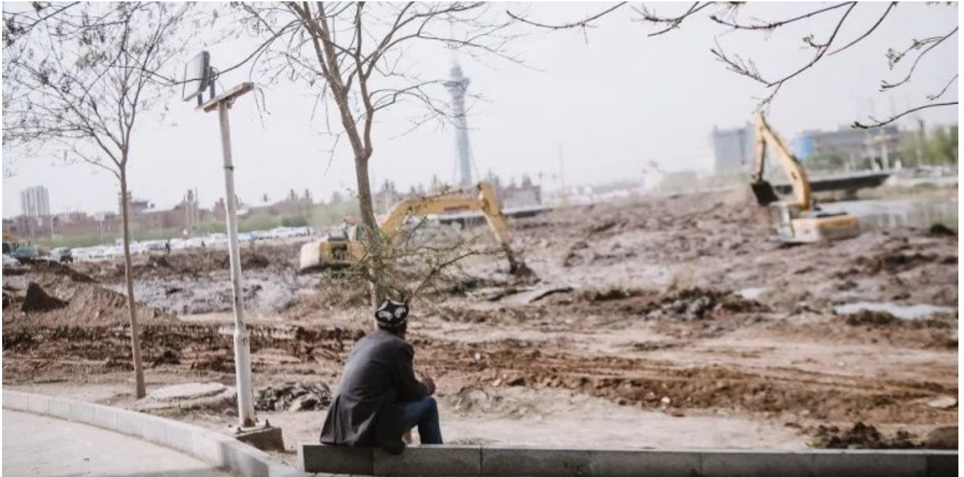
The meadow and the reed field in the photos above have now become a construction site (2018).
